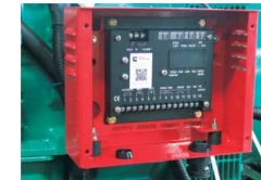
Speed Governor Installed externally for easy future upgrades
